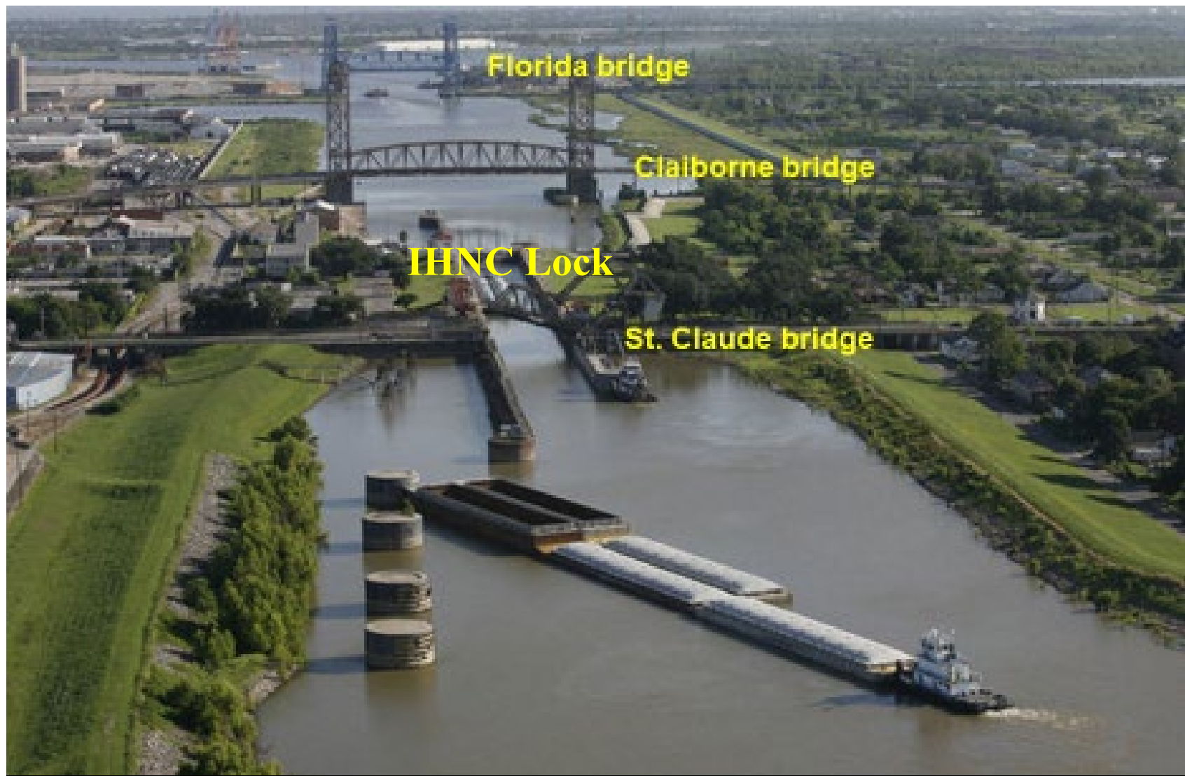
Figure 4: Looking North at IHNC Lock Complex
